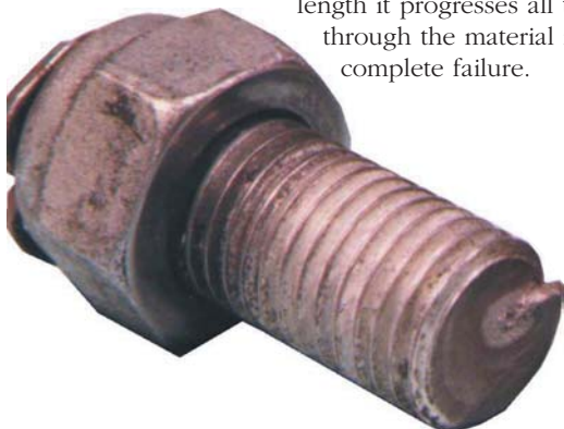
A fatigue crack can take years to progress through a bolt
